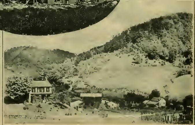
Residence of Chas. Brombacher, Mabert Ave.
